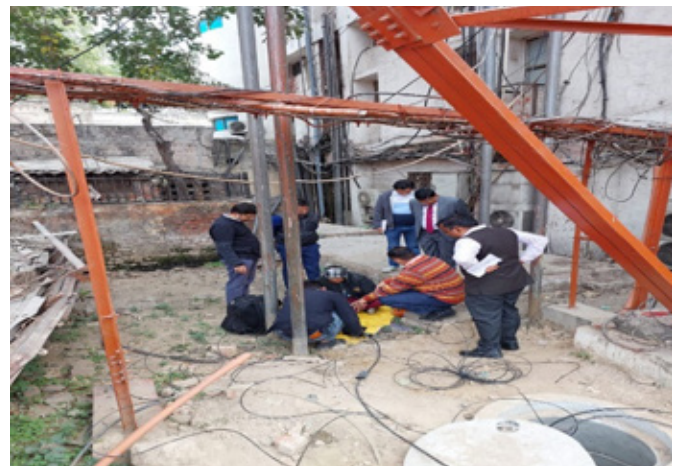
Inspection at Thomson Road, New Delhi
