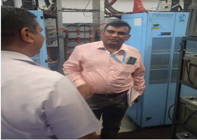
Inspection at Mahalaxmi PoP, Mumbai
