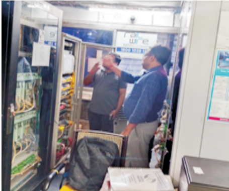
Inspection at Varanasi POP
