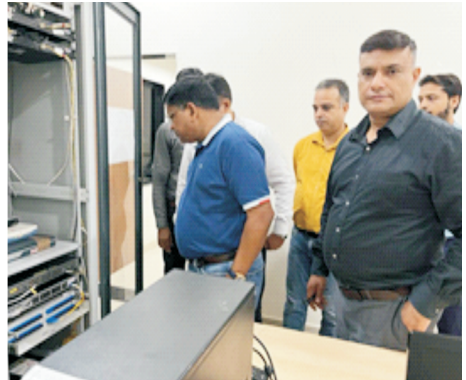
Inspection at Kevadia PoP
