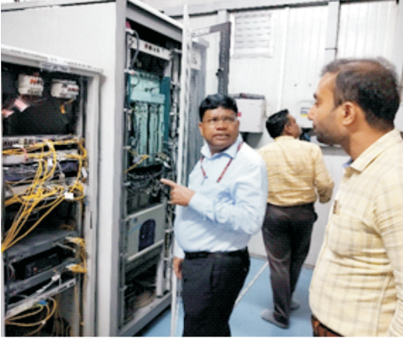
Inspection at Chandigarh PoP
