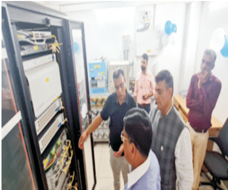
Inspection at Gandhigram PoP
